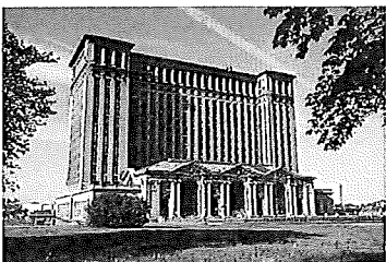
Before window re-installation (2010)
