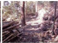
Improved path in bamboo grove
