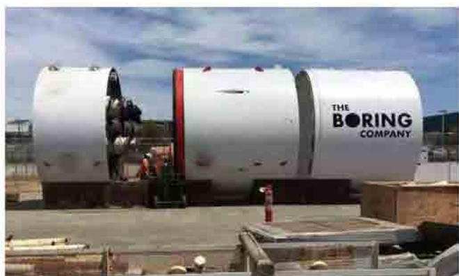
Musk's boring machine has already started tunnelling. Photograph: Instagram
