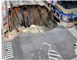
Huge Sinkhole Swallows Street In Fukuoka, Japan 28798 views
