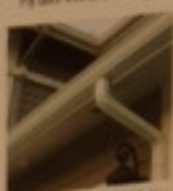
Downs, Downspouts and Gutters
