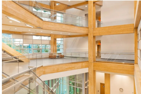
The Centre for Interactive Research on Sustainability, at the University of British Columbia, showing off some timber. | CIRIS
