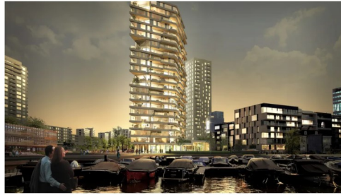
The Haut, the Netherlands' tallest wooden residential building | Arup
