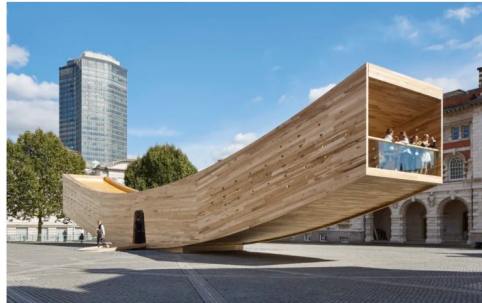
"The Smile," a public pavilion made of CLT, designed and built in London in 2016 by architect Alison Brooks. | Alison Brooks Architects
