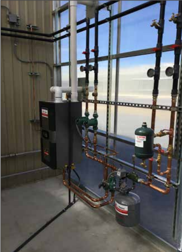
Raypak Boiler System
