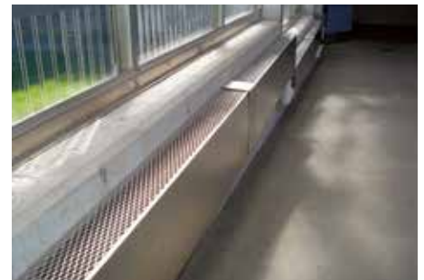
SunFin perimeter system in protective cover.
