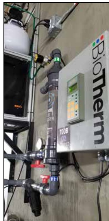
BioTherm's O2 Gen, The TOOB, and HANNA DO Meter working in tandem together.
