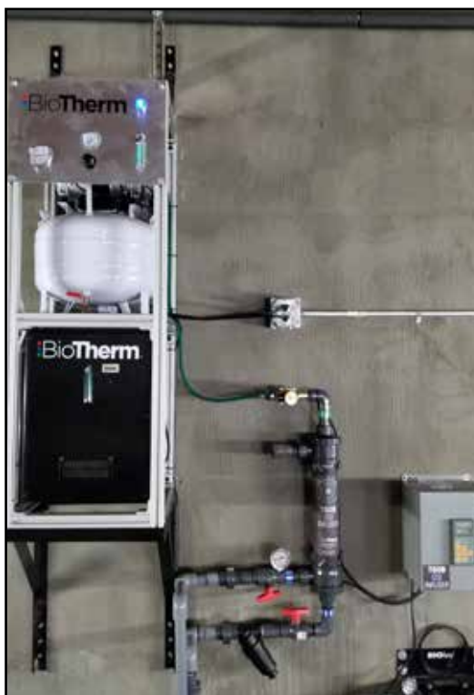
BioTherm's O2 Gen, The TOOB, and HANNA DO Meter working in tandem together.
