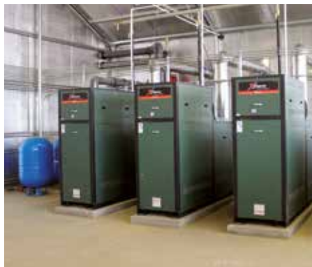
BioTherm grows with you so you can plan for the future. With a cascading boiler system, Raypak condensing boilers may be added as you expand.
