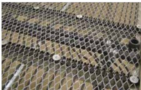
MicroClimate tubing provides even and consistent heat for Beth’s ornamental plugs.
