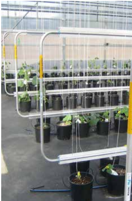
DuoFin heat pipe is strategically placed near the roots and in the canopy to provide gentle and stable heat.
