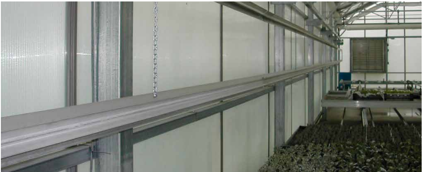
BioTherm's StarFin™ System lines the perimeter of this greenhouse.
