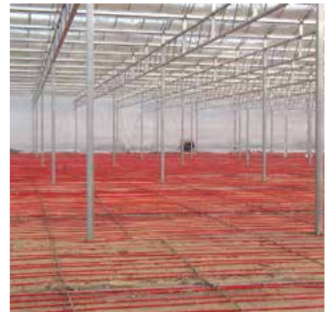
BioTherm HDX (high density extrusion) in-ground system provides an evenly heated surface for pots and flats.
