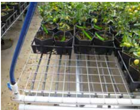
MegaTube around the containers provide direct and consistent heat to the root zone.
