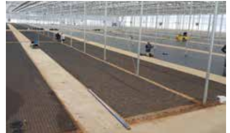
Michael’s BioTherm MicroClimate heated floor during installation
