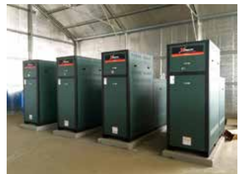
High-efficiency Raypak boilers (up to 95%).
