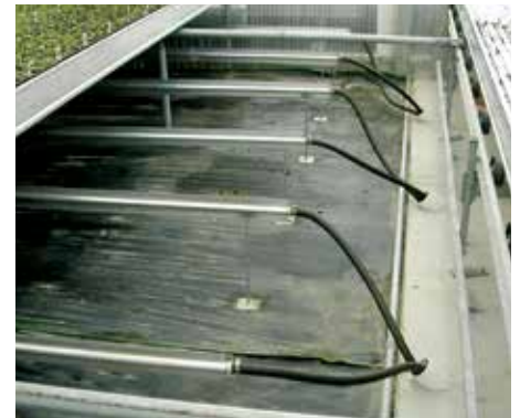
BioTherm DuoFin heat pipe provides an even and uniform heat, perfect for mobile benches.
