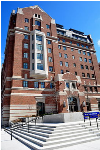
North Quad Residence Hall
