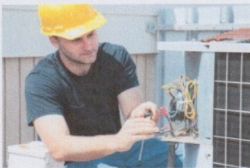
HVAC Repair Chicago
