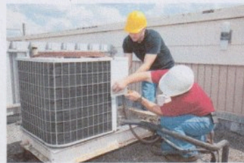
HVAC Installation Chicago
