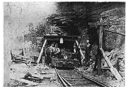
Entrance to mine shaft in West Virginia, photographed by Lewis Wickes Hine in 1908
