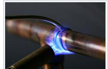
Soldering copper pipes using a propane torch and lead-free solder
