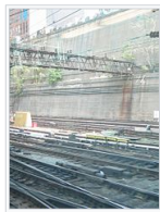
Track switches west of the station
