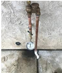
install water pressure regulato... quanterainc.co
