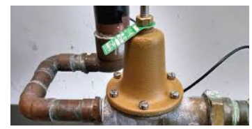
Water Pressure Regulator Installation ... greensplumbingco.com
