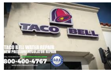
Taco Bell Water Pressure Regulator Repair sosplumbingroofer.com
