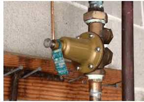
Water Pressure Regulator Repair ... johnselectricservice.com
