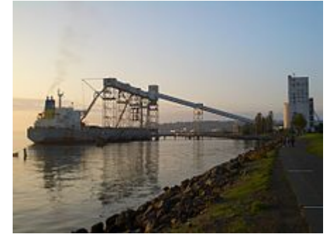
A boat being loaded at Pier 86 Grain Terminal in Seattle
