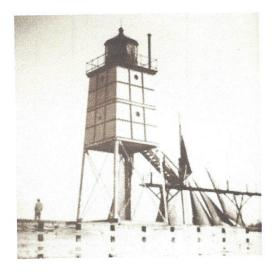
The Original lighthouse built at the Holland Harbor location was a small, square wooden structure built in 1872. In 1880 the Lighthouse Service installed a new light atop a metal pole in a protective cage. The old lantern was lowered by pulleys for service.
