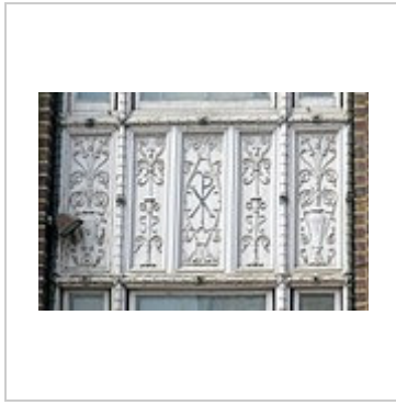
Chi-Rho on YMCA building, Over-the-Rhine , Cincinnati , Ohio .
