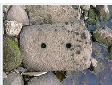
A typical stone railway sleeper
