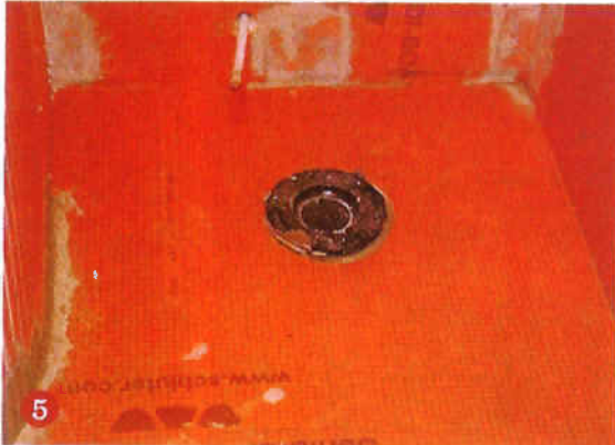
5. Kerdi-Board surrounds the toilet flange and acts as a barrier between the concrete slab and the radiant heat wires
