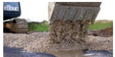
Aggregate placed on top of TriAx geogrid prior to full compaction.
