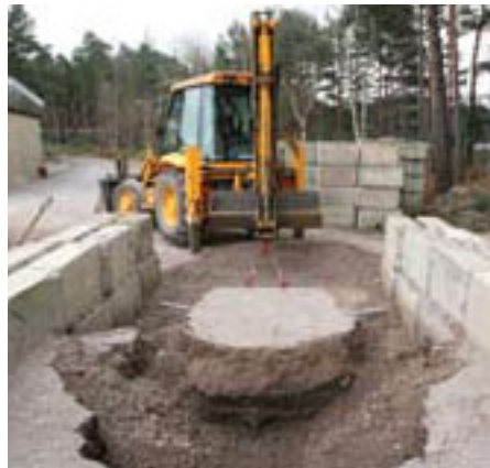
Excavation of TriAx for installation damage tests.
