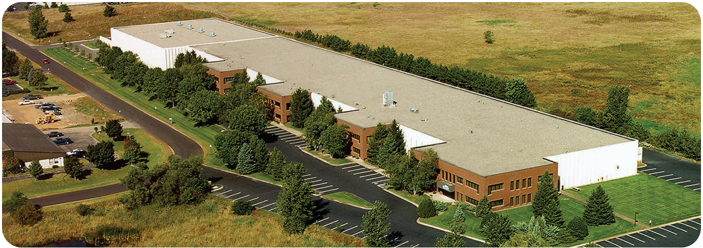
Cat Pumps occupies over 145,000 sq. ft. at its world headquarters in Minneapolis, MN.
