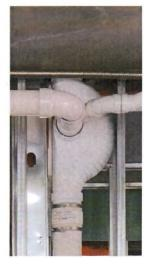
We recommend using E-Z Flex couplings on fab openings 3" or larger. They can also be used on the 2" fab openings.
