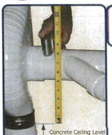
Make sure all the fabricated overhead piping will fit into the drop ceiling space. The stack sleeve can be raised up to recess the stack up into the slab if necessary. Drop ceilings are usually 12". Here we are 7-3/4" below the concrete ceiling.
