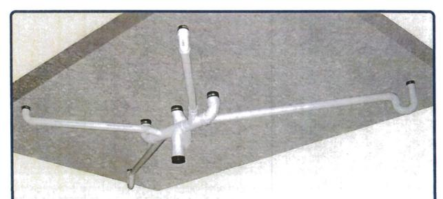
The embedded sleeve couplings also act as a hanger and riser clamp (see WH listing) for the horizontal and vertical piping. Additional hangers may be required if the branch piping exceeds the horizontal lengths allowed by code.
