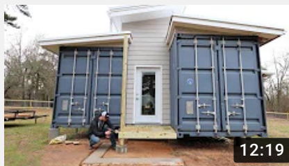
Building The Front Entry For Our HOME!
