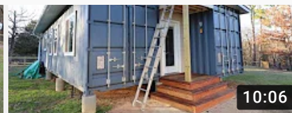
Building An Overhang For Our Front Porch!
