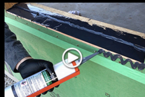
Check out this European Window Installation With Liquid Flash
