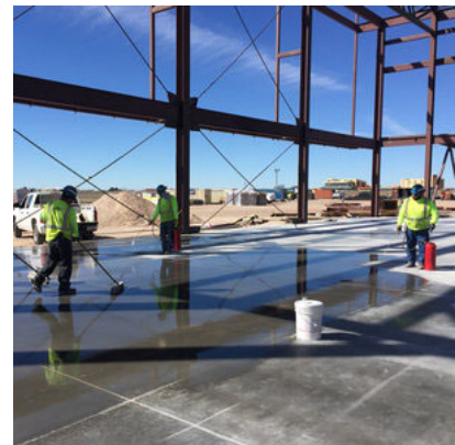
Creteseal CS2000™ being applied for a retail center.
