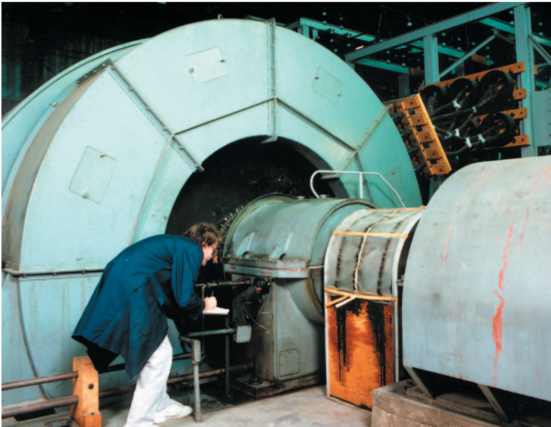
High-power 762 MVA short circuit test generator.
