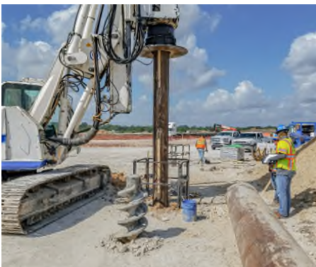
Drilled Pier Drilling
