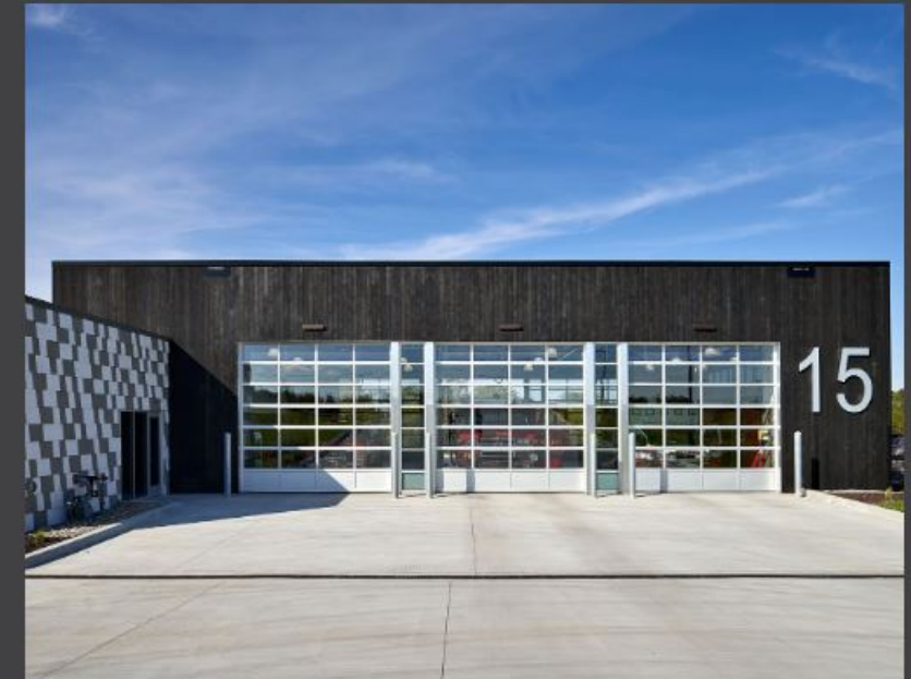
KCMO Fire Station 15
