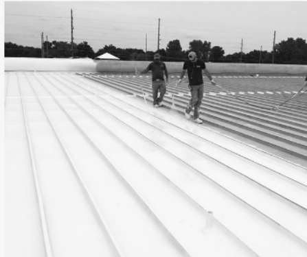
Safe Harbor Commercial Roofing
