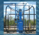
The **QuickSander**™ is a high-performance sand-dispensing system that can be installed on service track and mainline operations.
