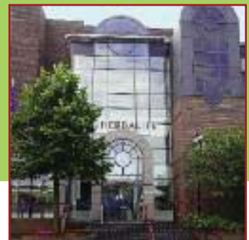
U.K. Distribution Center
