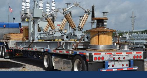
DIS-TRAN's XPS arrives fully pre-assembled, in one easy delivery, ready to be installed and energized.
