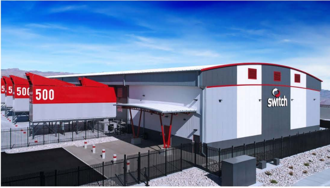
Switch SMART Research & Development Center / Switch LAS VEGAS 12 Data Center – A Switch MOD 100 Facility The Core Campus, Las Vegas, Nevada, USA
